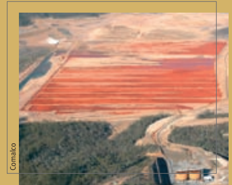
Waste from the alumina refinery is pumped to a residue management area before being rolled, compacted and dried
